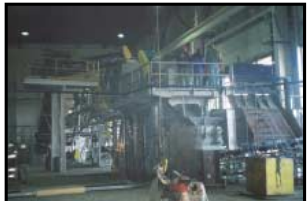
“Washery Installation Began September 2002”
