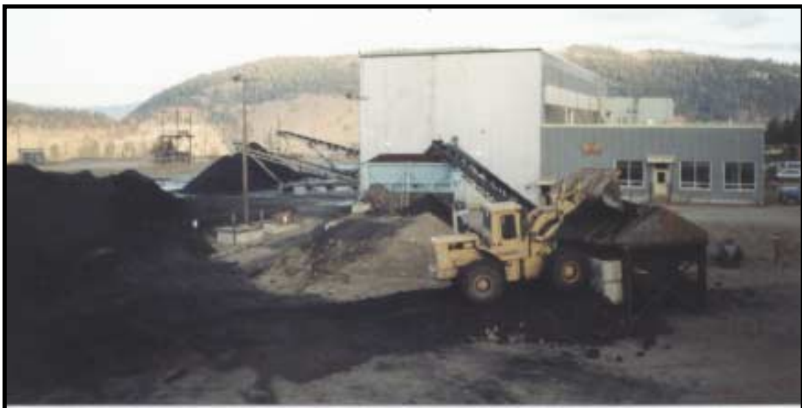
“Wash Plant completed and First Production in November 2002”
