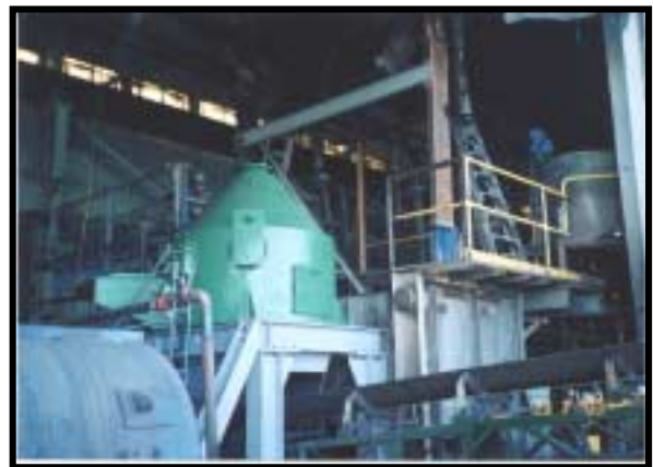
“Dewatering Centrifuge Installation 2003”
