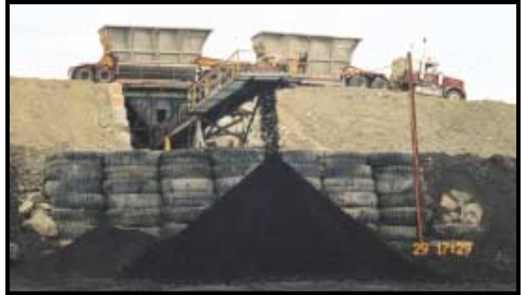
“New Truck Dump Facility Built by Compliance during the 2003 year”
